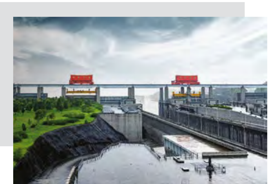
Three Gorges Dam, China
